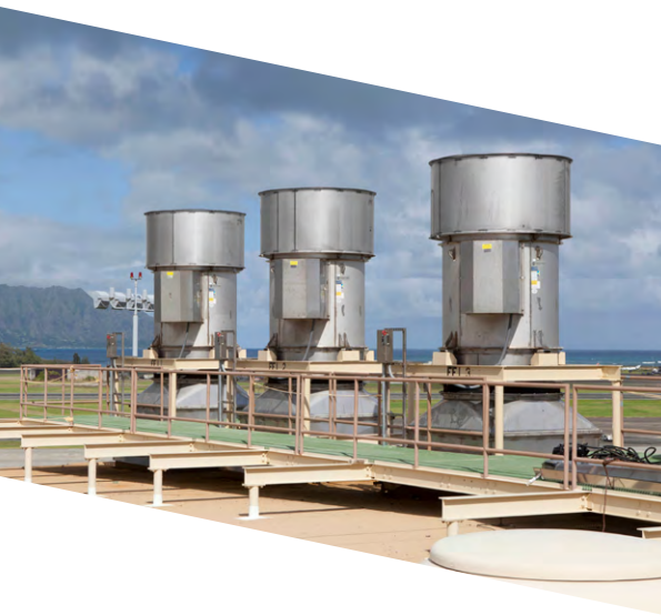
Model TCVX Vaneaxial Fan with Adjustable Pitch Blades
