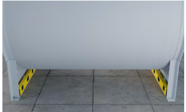
Carefully level the fan on the foundation
